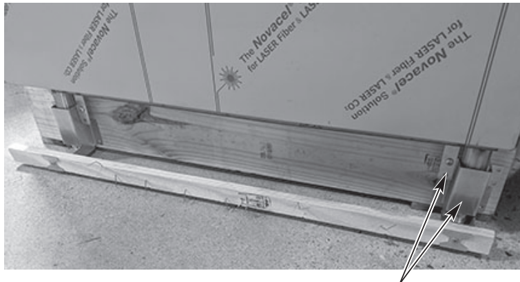
REMOVE SHIPPING BRACKETS (4 LOCATIONS)
