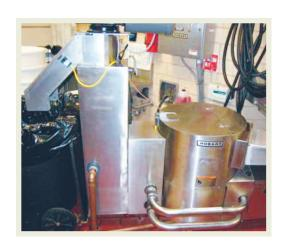
After installing the new Hobart system in 2007, the amount of solid waste has decreased significantly. The waste was reduced from 300 gallons (15 loads of a 20-gallon trash container) to a single 64-gallon toter. The physical strain is also lessened because the toter is wheeled to the waste collection site. Prior to switching to the Hobart system, Gettsyburg College hired an outside refuse collector to transport the solid waste produced by Dining Services.
