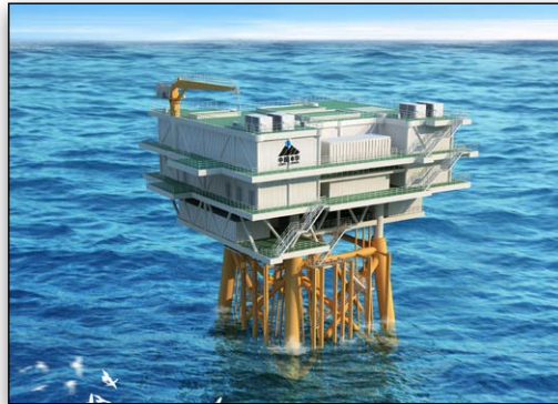
Bentley OpenWindPower was used to design a range of foundations, for wind turbines and offshore substation in water depths that range from 2.6 meters to 20.5 meters.
