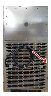
Close louver door remove rear condensing unit cover and check if glycol ball valve is in the open position. Re-attach rear louver.
